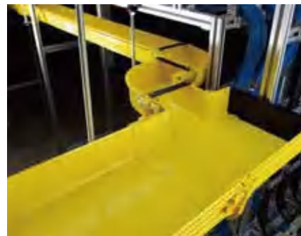
光纤槽道水平弯头及出口 Optical fiber channel horizontal elbow and outlet
