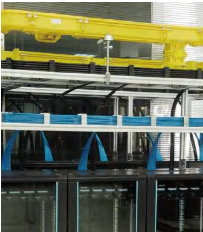
机房走线架机柜顶部安装方式 Cable rack installed on top of machine cabinet
