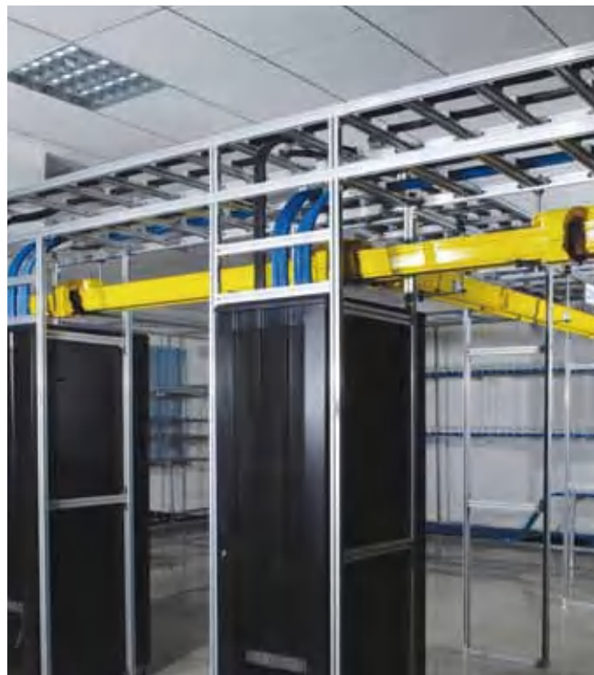
机房式走线架地面支撑安装方式 Ground support installation for cable rack in machine room
