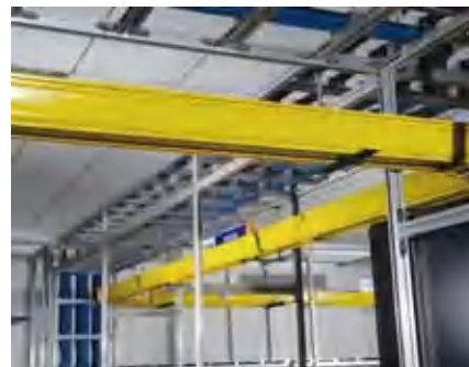
机房式走线架地面支撑安装方式 Ground support installation
